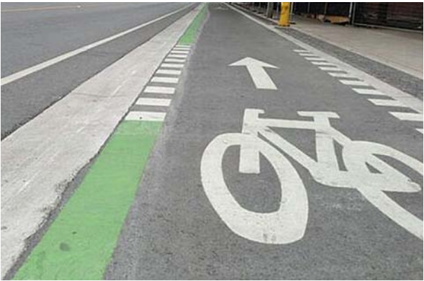
Bike Lane Delineation and Symbol Marking
