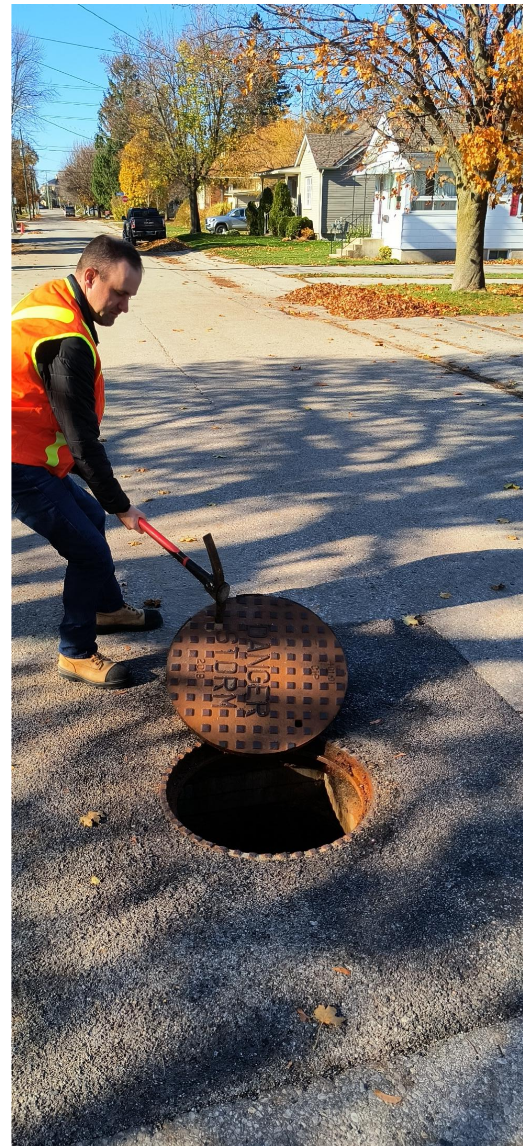
Remove maintenance hole lid
